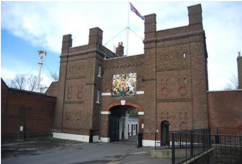
Dockyard Main Gate
